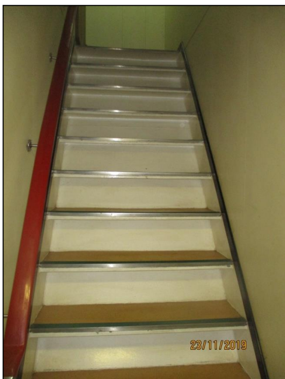
Figure 3: Section of the stairway, seen from the bottom (poop deck level)
