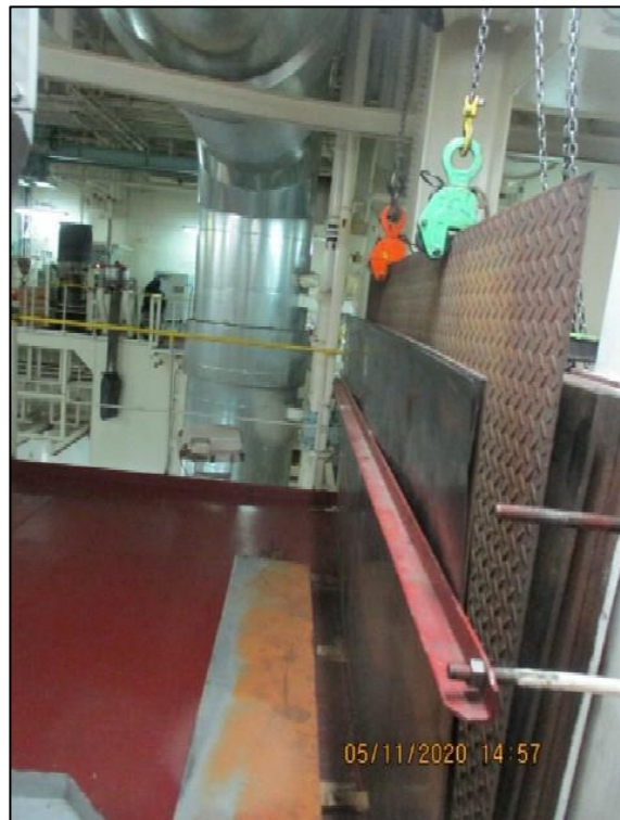
Figure 10: Extraction of a steel plate using the lifting clamps
