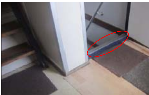
Figure 3: The lower horizontal part of the door frame
