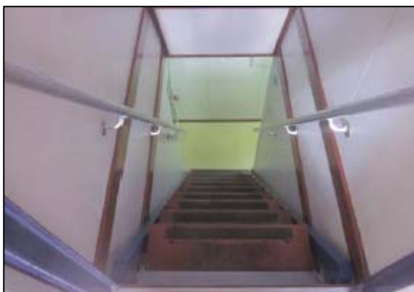
Figure 1: The AB was found lying down at the bottom of this staircase
