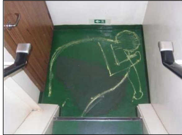
Figure 4: The bottom end of the stairway where the injured crew member was found
