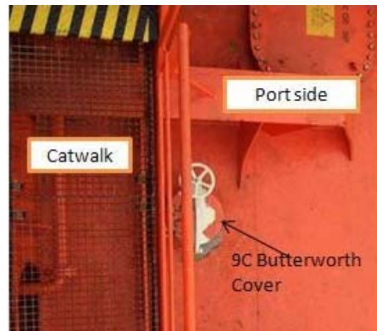
Figure 4: View of no. 9 centre tank Butterworth cover from the catwalk
